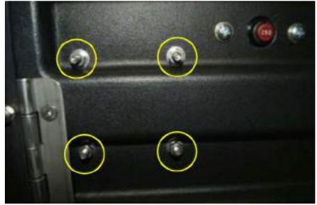
Step 6: Connect the short red 4-gauge cable marked “right side circuit breaker” from the 1-2 Switch to the right side of the circuit breaker (toward door), install the nut, and tighten.
