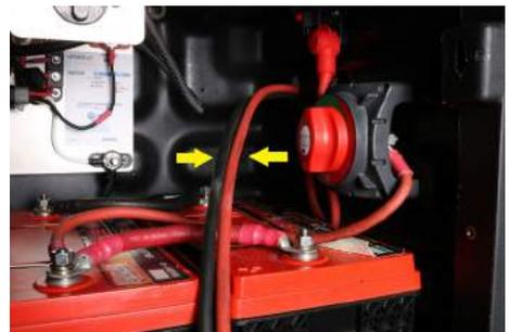
Step 17: Pull the 4-gauge red and black cables back out of the battery box so it is easier to work on them. Cut off the excess.
