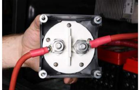
**Step 3:** Mount the 1-2 Switch using the provided hardware.
