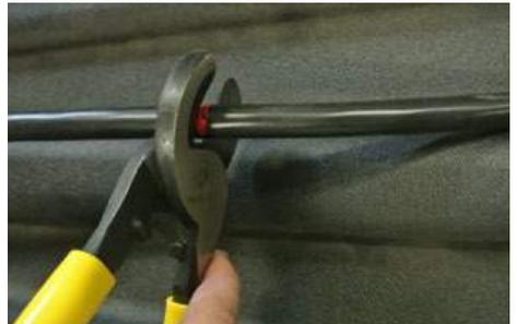
Step 6: Cut about 8 inches off of the conductor.
