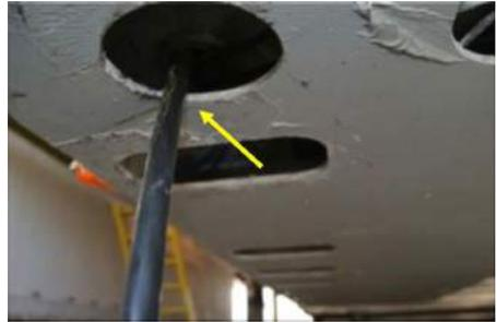
Place the cable clamps along the 4-conductor jacketed wire every 6 inches to ensure proper support for the cable. Avoid sharp edges and possible chaffing points.
