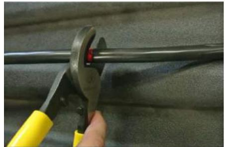
**Step 6:** Cut about 8 inches off the jacketed portion off the conductor.
